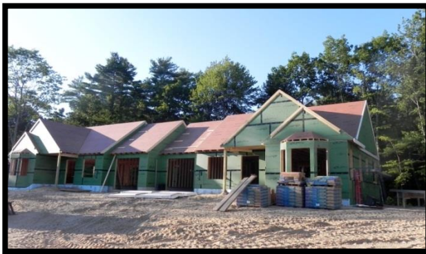
Duplex under construction at Wesley by the Sea
